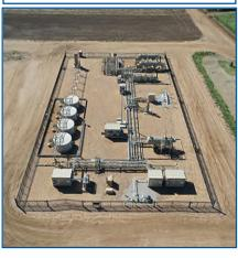
Production facilities are constructed adjacent to the wells to collect and separate the oil, natural gas, and water that are produced. Facility production is 30-45 days of work, completed in stages over about four months.
