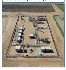
constructed adjacent to the wells to collect and separate the oil, natural gas, and water that are produced. Facility production is 30-45 days of work, completed in stages over about four months.
