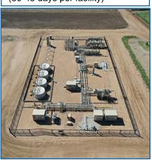
facilities are constructed adjacent to the wells to collect and separate the oil, natural gas, and water that are produced. Facility production is 30-45 days of work, completed in stages over about four months.
